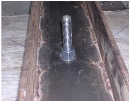
Figure 4.28: HAS-E anchor after installation
