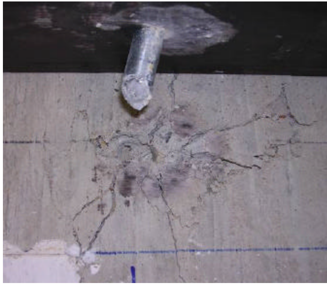
Figure 5.45: Failed Specimen WEDGB40
