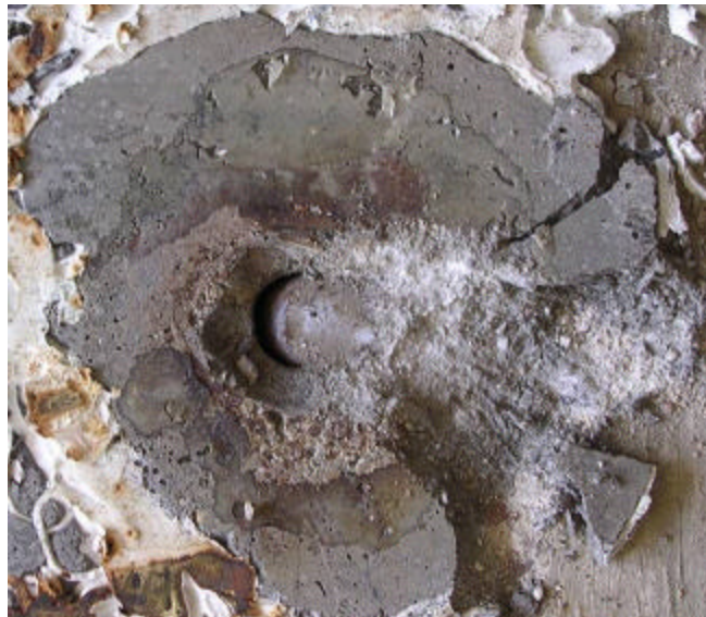
Figure 5.10: Crushing of grout in front of stud (Specimen POSST-ST(F))
