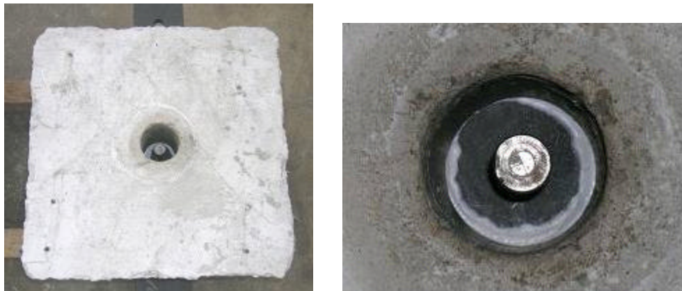
Figure 4.25: Precast hole with welded stud before grouting
