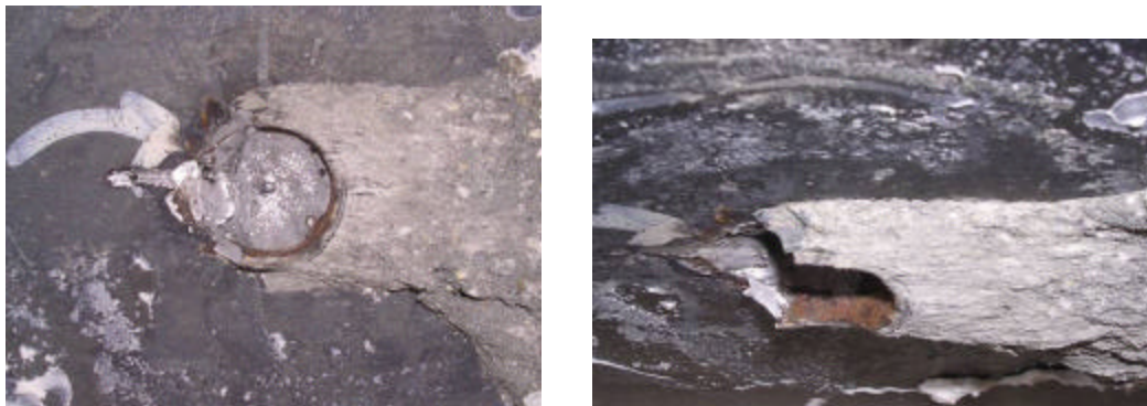
Figure 5.6: Failure of weld in shear (Specimen POSST-ST)
