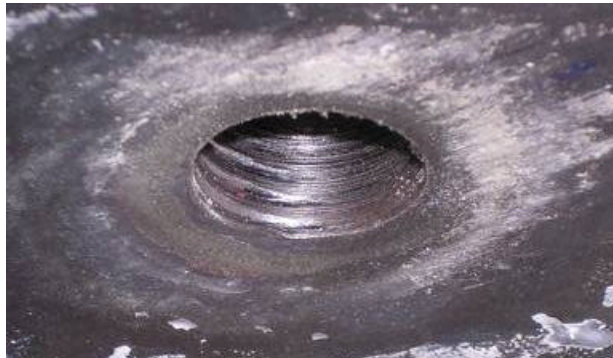
Figure 5.14: Bearing deformation in steel plate (Specimen DBLNB-ST)
