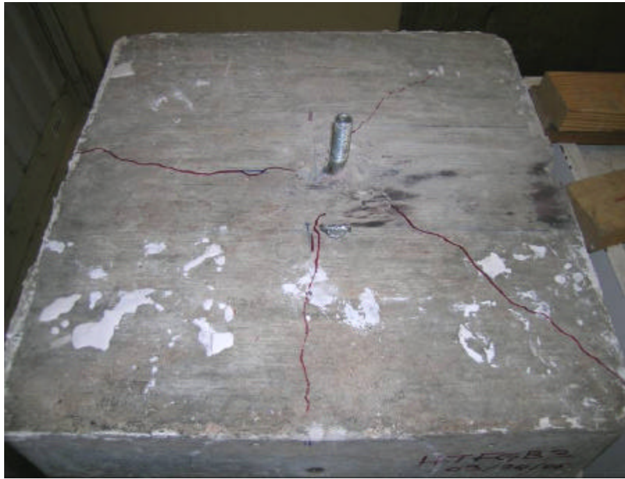
Figure D.7: Concrete failure of Specimen HTFGB3
