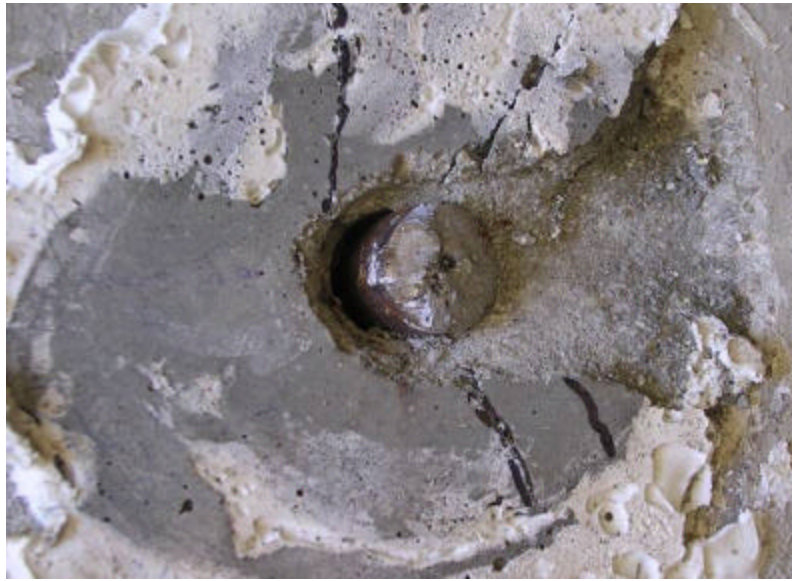
Figure 5.7: Crushing of grout in front of stud (Specimen POSST-ST)
