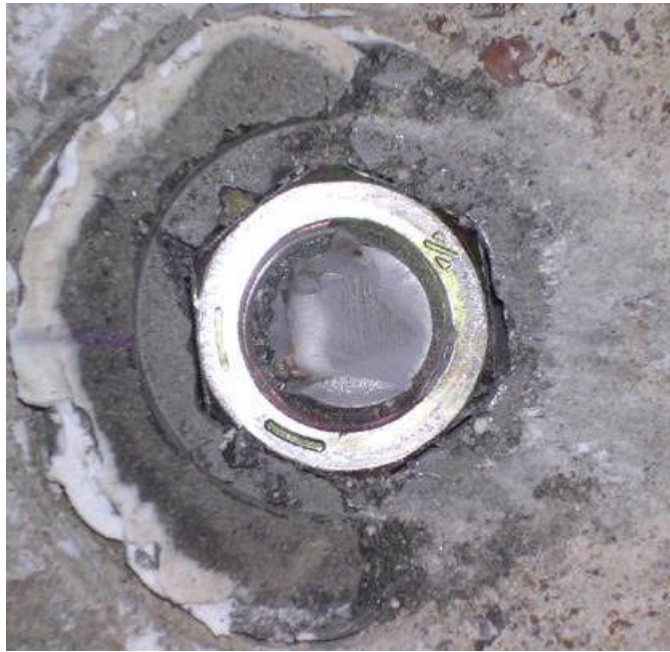
Figure 5.12: Failed connector at steel-concrete interface (Specimen DBLNB-ST)
